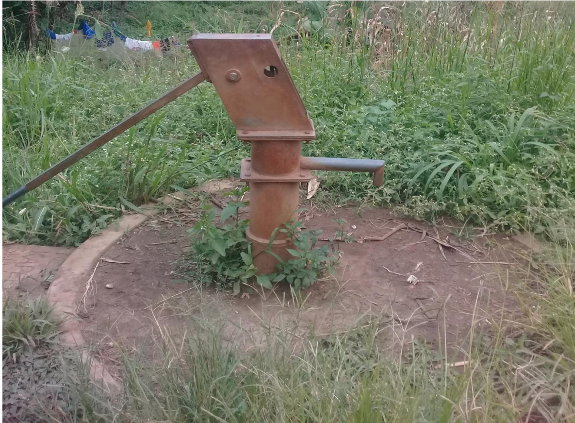
Plate 3: A dry borehole at Kapeeka Village. Source: Field survey 2017
