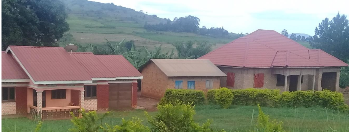
Plate 5: Permanent houses in Kadukulu Village Nyabyeya Parish. Source: Field survey 2017
