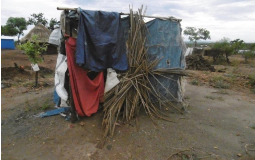
Plate 1. A pit latrine with shields made out of papyrus and old tarpaulins that work as a temporary wall
