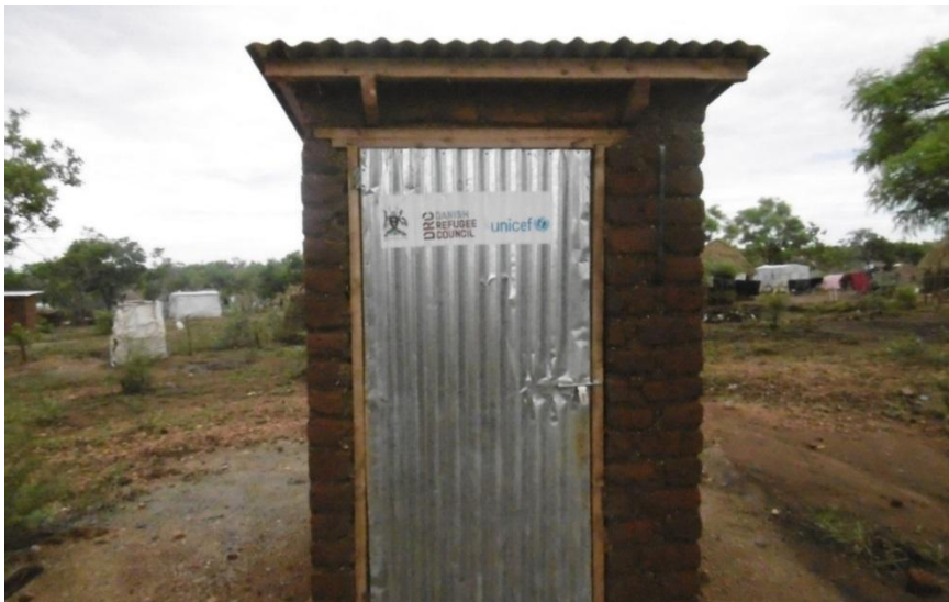
Plate 2. A pit latrine with walls made out of bricks and cement as recommended by Sphere Minimum Standards (C) 2017
