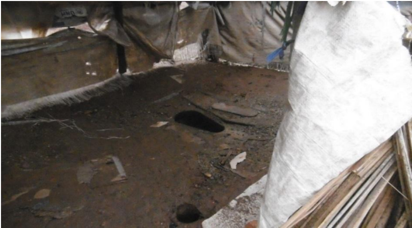
Plate 3. A pit latrine with temporally screens which work as walls and does not have a covering lid. (C) 2017
