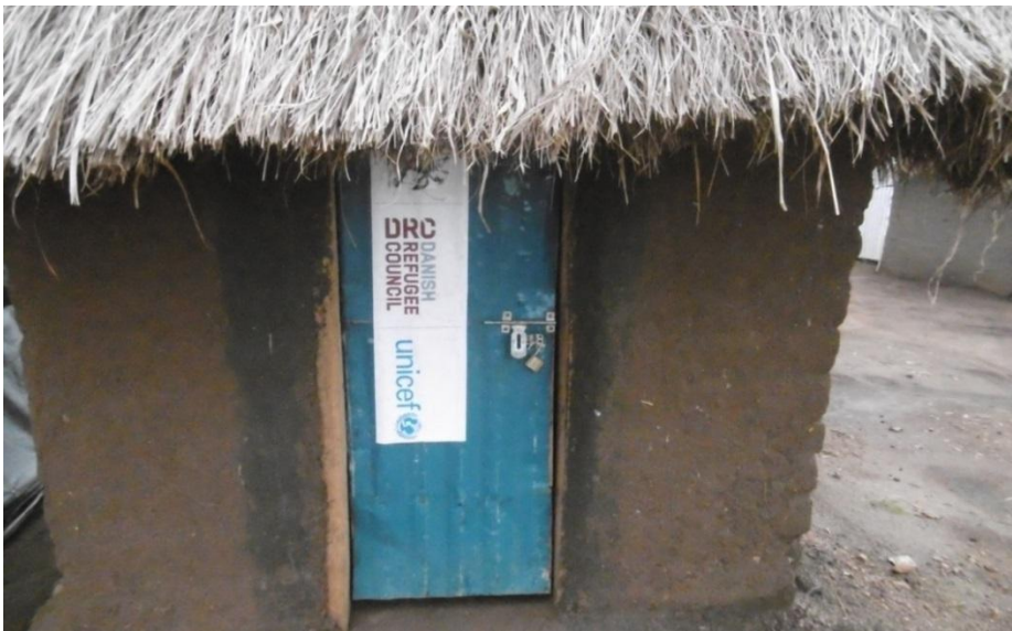
Plate 4. Pit latrine roofed using grass and it is lockable (C) 2017
